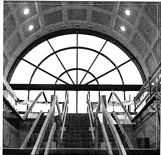
Ornamental Steel – Plattsburgh International Airport
