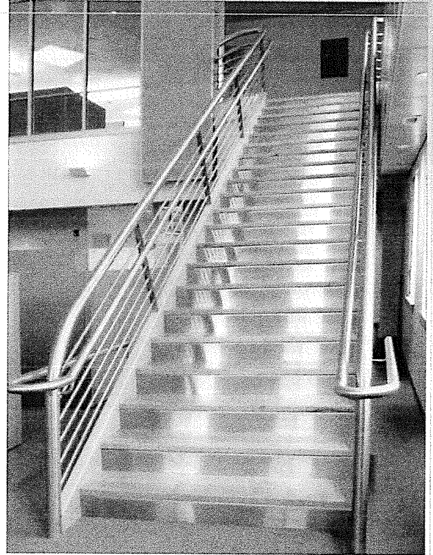
Infineon Office Stair & Railing System
