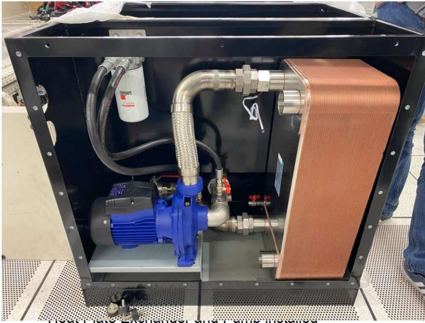
Heat rate Exchanger and Pump installed
